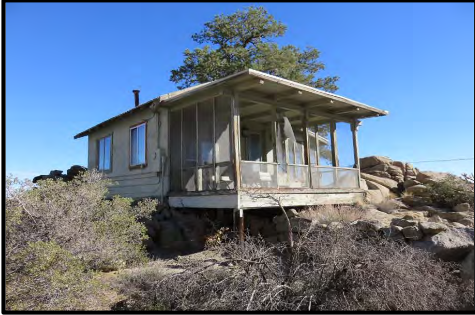
The building identified as the “guest quarters” and called “The Roost” by the Shumway’s
